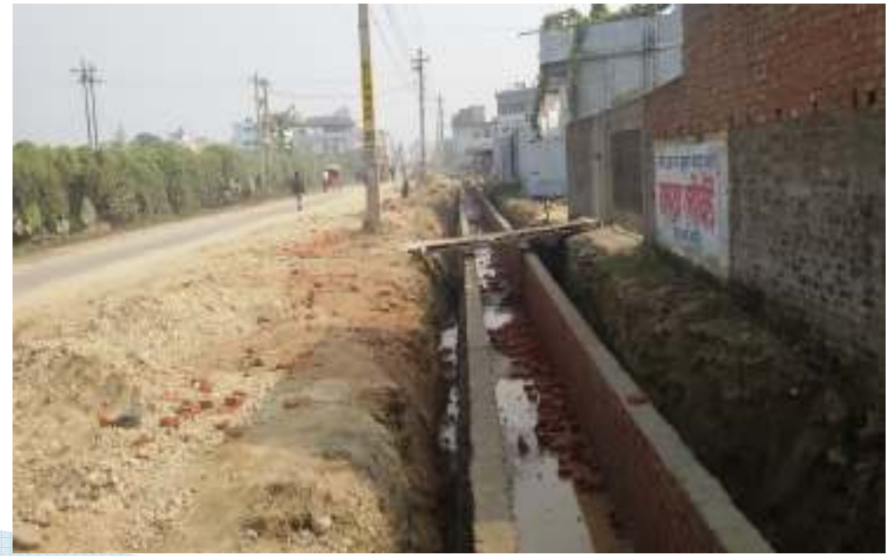
RCC Drain work at 1 st By Pass Road and B/W at Railway Road
