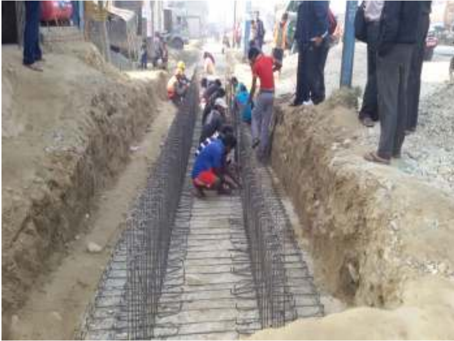
RCC Drain work at 1 st By Pass Road and B/W at Railway Road
