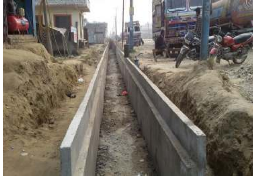
RCC Drain work at 1 st By Pass Road and B/W at Railway Road
