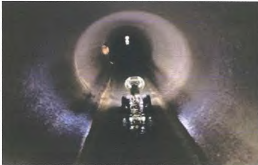
Figure 13: Sewer line inspection by CCTV
