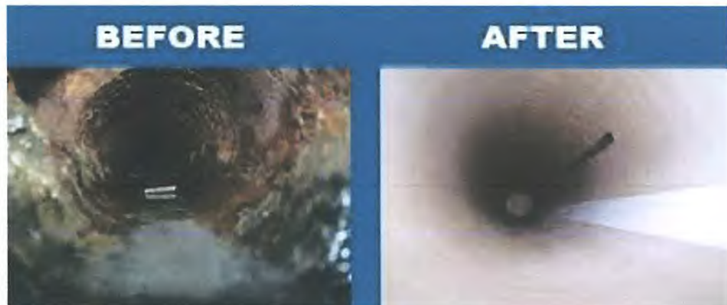
Figure 2: results of hi-velocity cleaning of sewer
